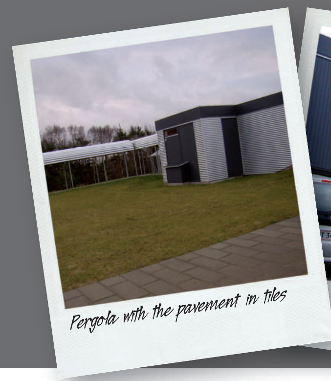
2030m² administrative building with big office, toilets and connecting passageway arranged in 47 modules
